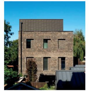
I deliberately chose Wasserstrich linea 6012 from Vande Moortel which I discovered a few years when the bricks were used for a project in London. It was the first time that I had seen this type of facing brick and I liked the clean lines where the facing brick is brought into focus by the use of raked mortar. I knew that was what I wanted for Brickfields too."
