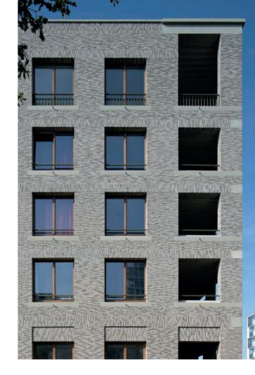
Hama combined these two Linea facing bricks with a transparent green glazed brick which has also been used in the communal entrance halls and interior spaces. Like the facing bricks, the glazed bricks also have a Wasserstrich texture which is still clearly visible through the transparent glaze. This creates an extremely lively surface in terms of the glazing and colour variation.
